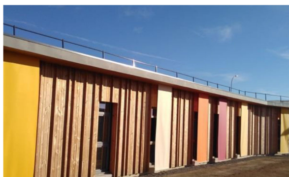
AIST 87 - construction HQE © Sébastien Rogala
